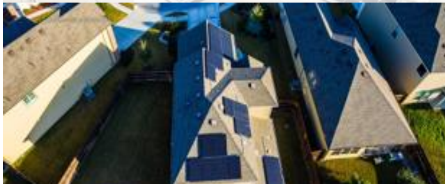
5 kW-10 kW, Residential roof
